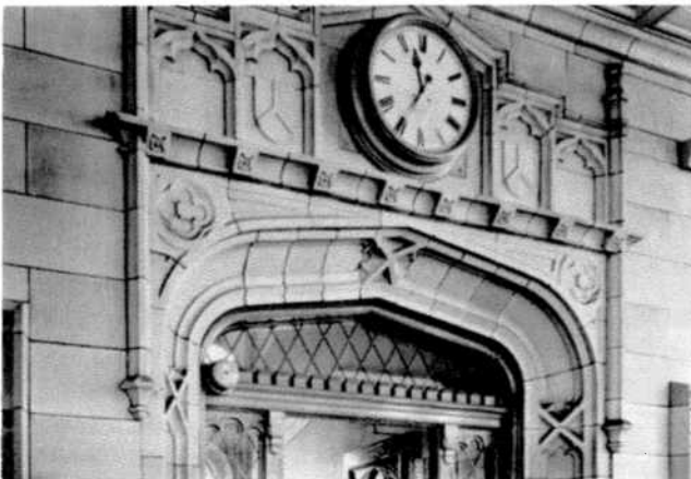
The very fine glazed terra-cotta interior of the Pumping Station dates from the early 1900s. (Bob Thall, photographer)
